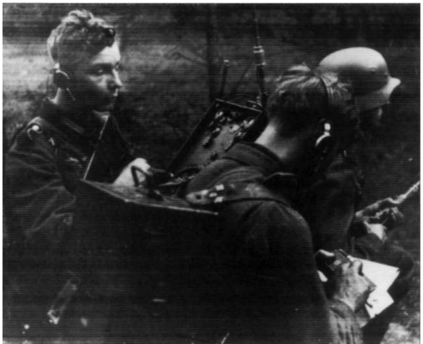
German Pack Wireless Type d2 for company-battalion-regiment communications. Radios gave the Germans an advantage in command and control. During all of Barbarossa they captured only
